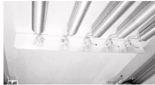
Figure 3: Springs hooked downward
